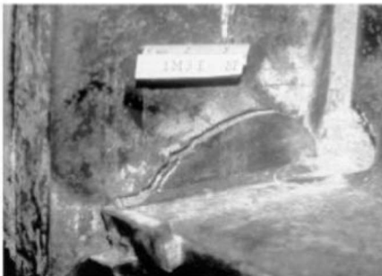
(b) Beam bottom flange weld fracture causing a column direct fracture
