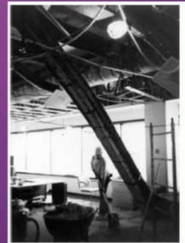
Figure 12-11. Example of brace buckling – October 1, 1987 Winter earthquake
