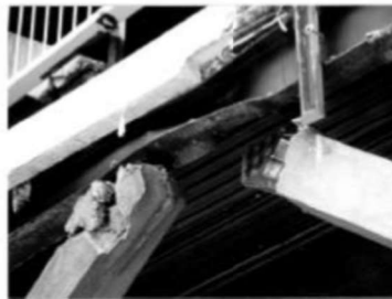
(b) Severe distortion of beam without lateral support at location of channel braces
