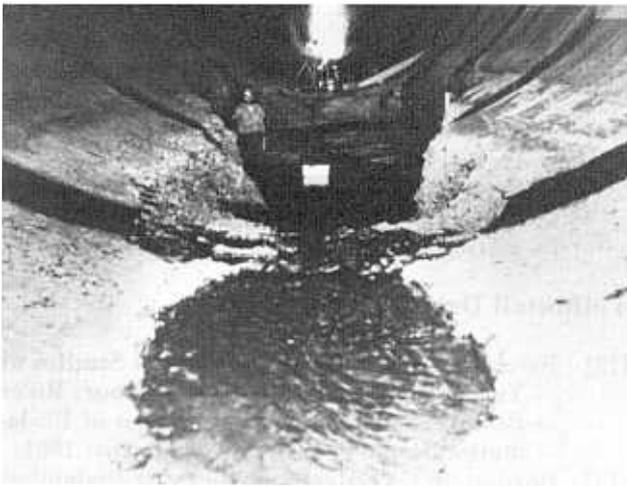
FIGURE 7-13.— Yellowtail Dam, tunnel spillway — major damage downstream of elbow.
