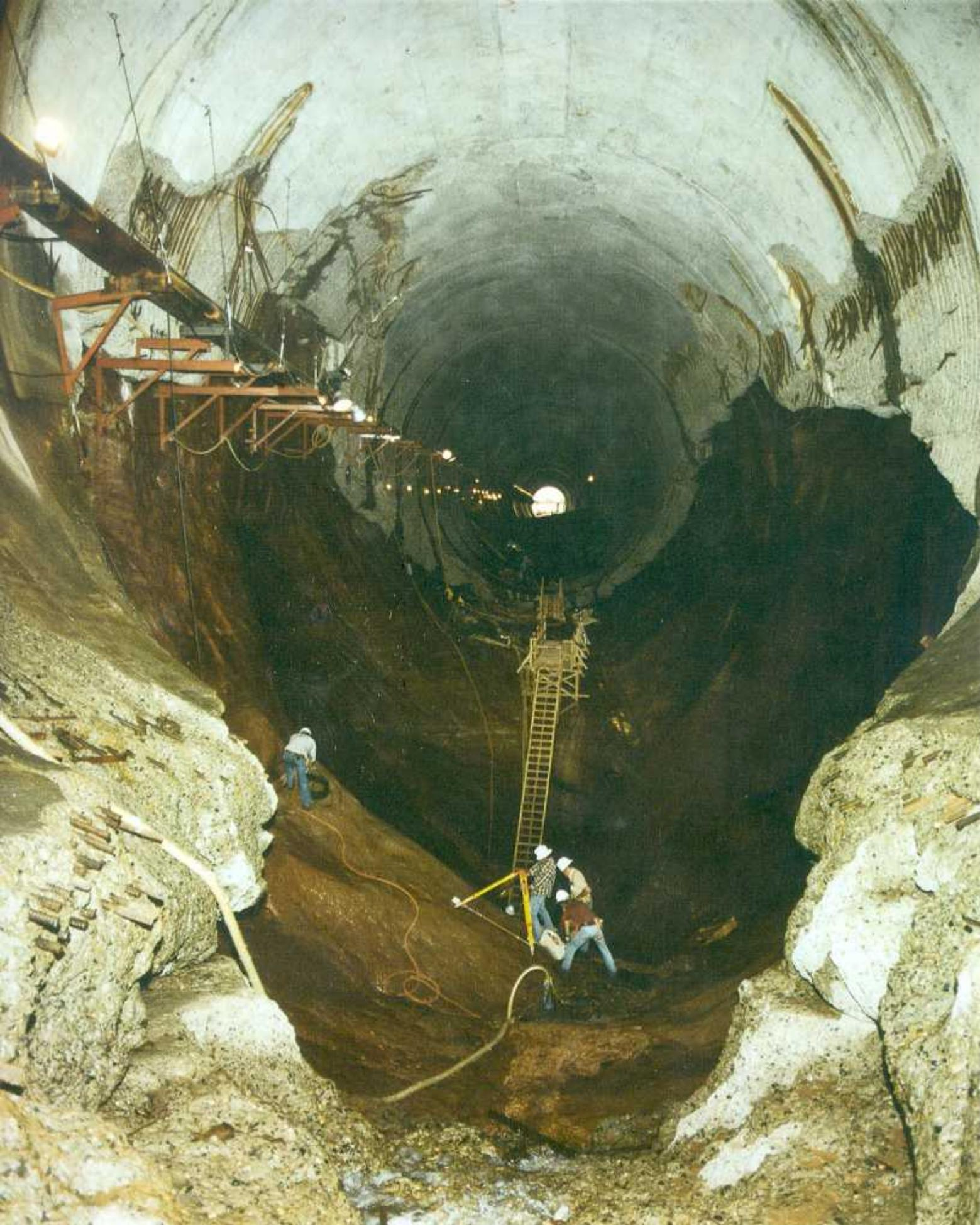
**FRONTISPIECE.**—Glen Canyon Dam. Left Spillway Tunnel Sept. 1983. The “big hole” in the spillway invert was 11 meters deep. Photo C557-400-690NA
