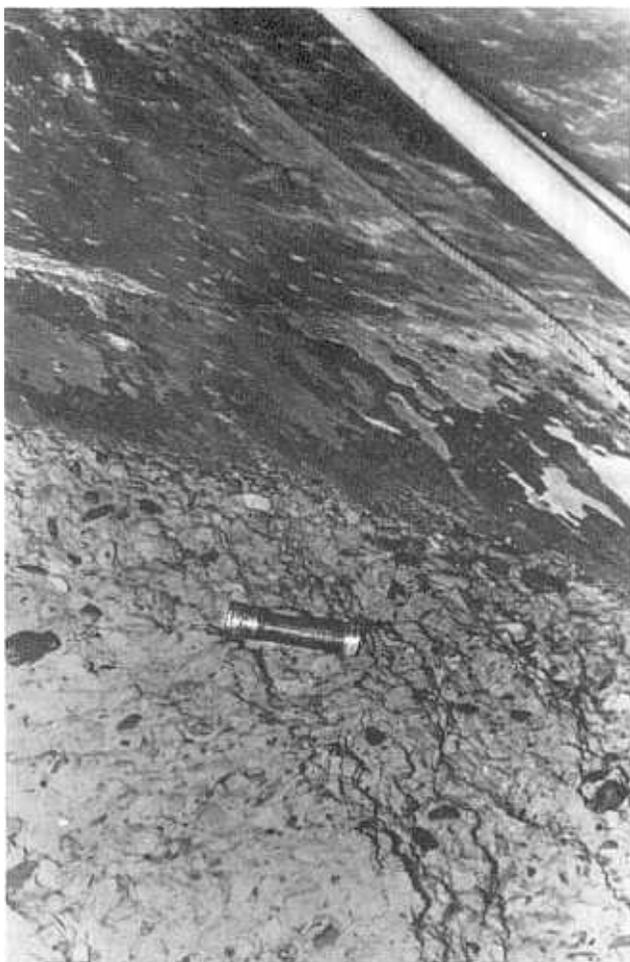
FIGURE 7-8.—Hoover Dam, Arizona tunnel spillway — misalignment that caused major damage.
